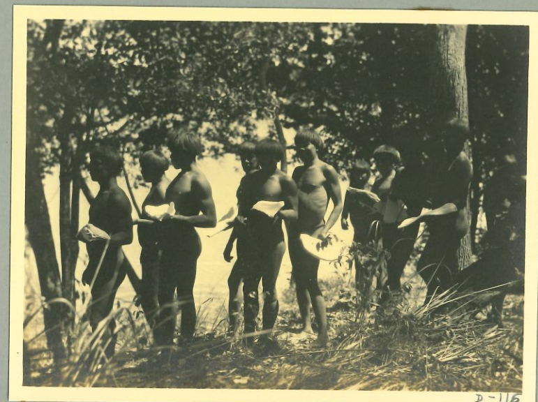
D-116 Bringing presents of Bread - junction 7 th de Sept. River + Caluene Neg. 27613
