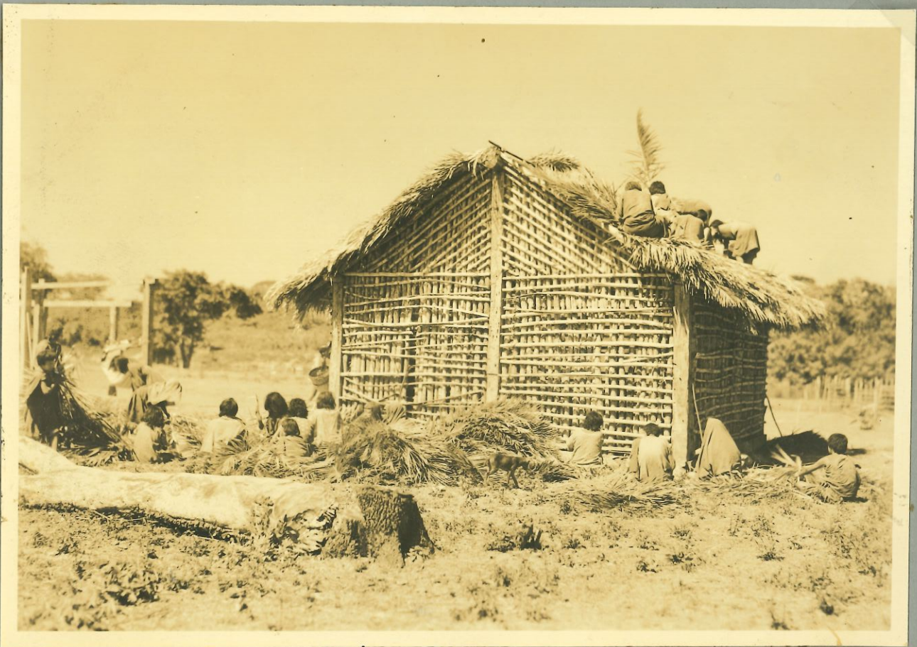
A-147. Bororo Building hut
