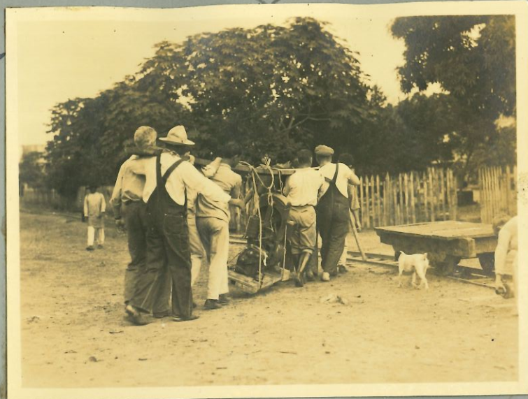
23A - Moving Expedition Kobler lighting plant at Desobrocks Neg. 27345
