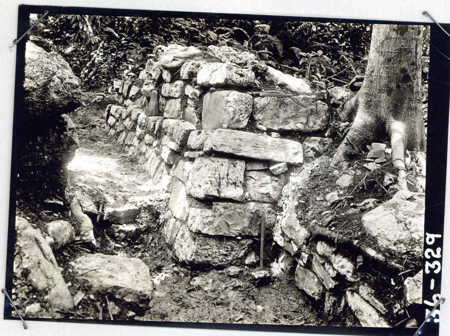
Fig. 3 Right front corner and end of building platform and building of Str. S-17; at the observers right, right end of Unit C of Str. S-17.
