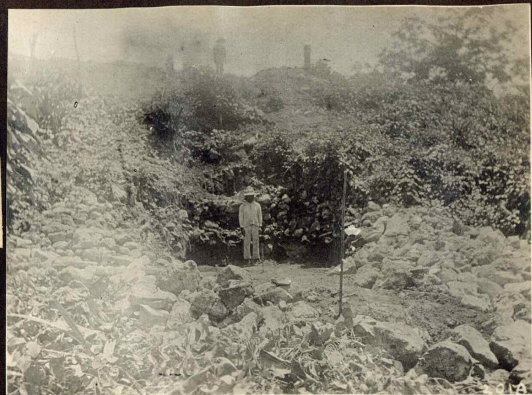
No. 13. Chama. View of the bottom digging
