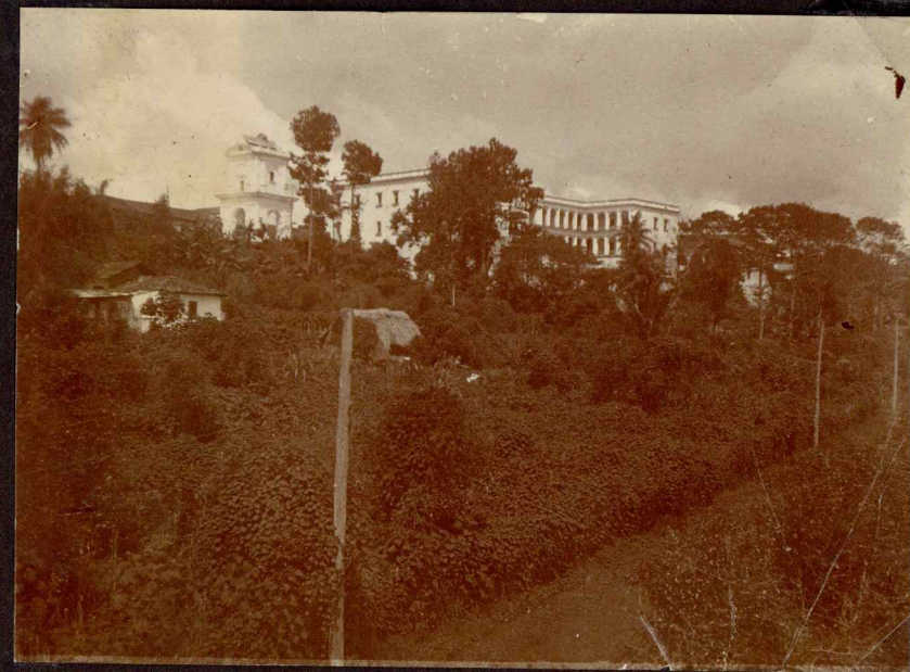
No. 6. A View of the government buildings in Coban
