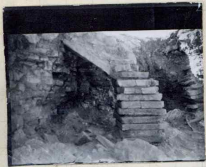
9. north bath of caldarium
