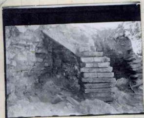
10. north bath of caldarium
