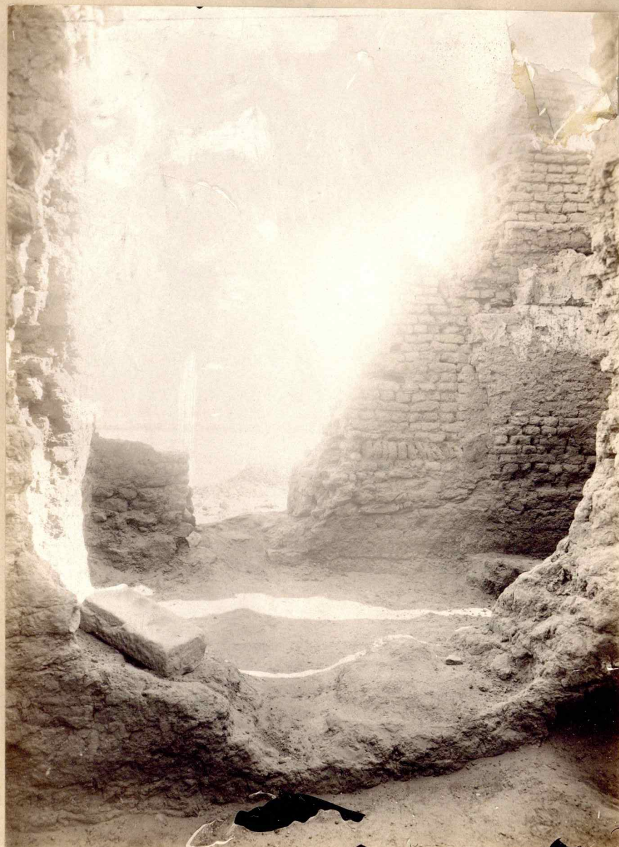
The Castle; the restored gateway seen from inside
