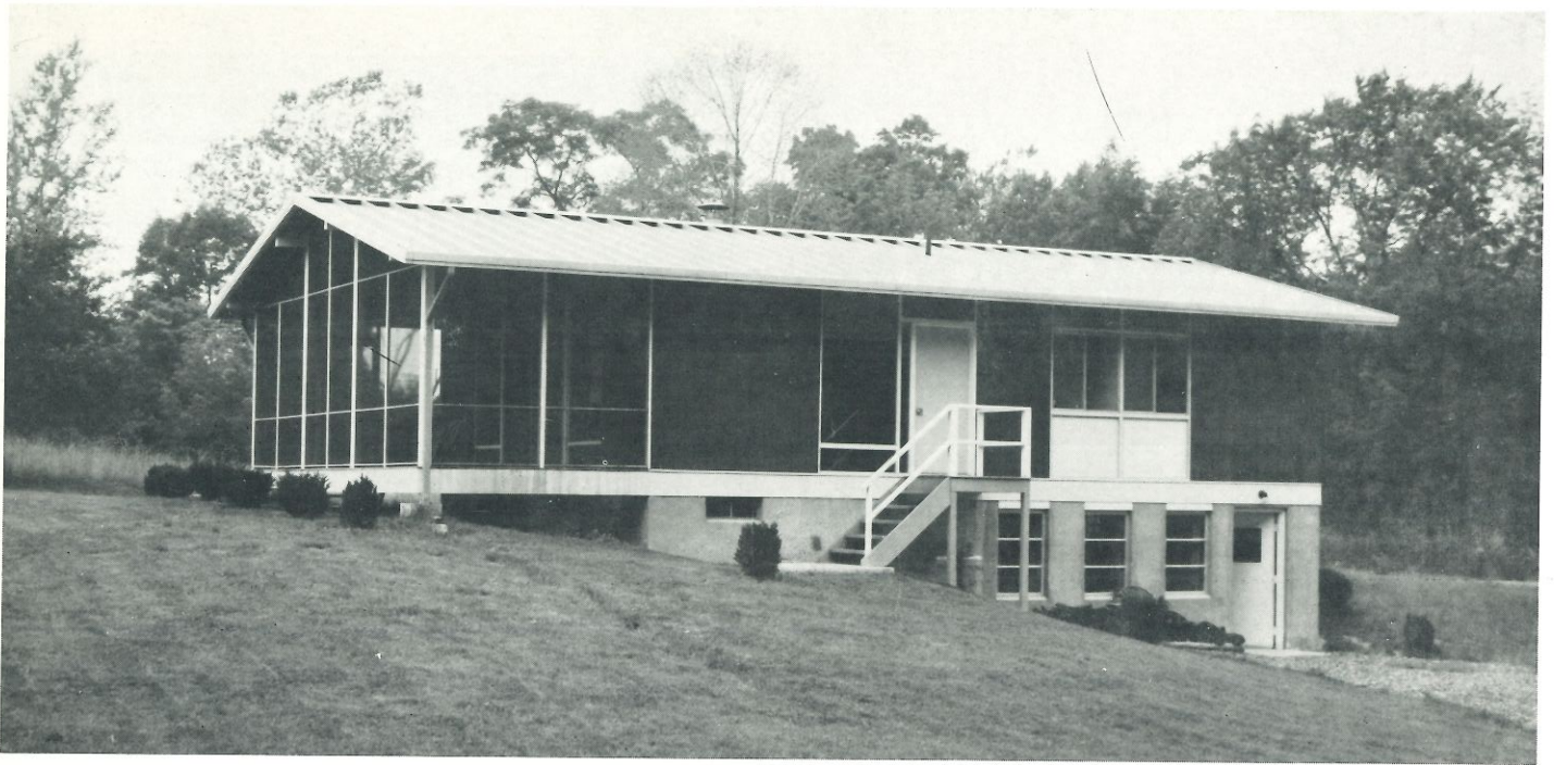
The new office building at the Harvard Black Rock Forest with living quarters on the upper level.
