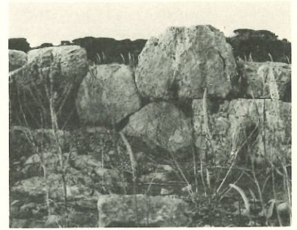
Figure 18. A section of the walls on the west side.
