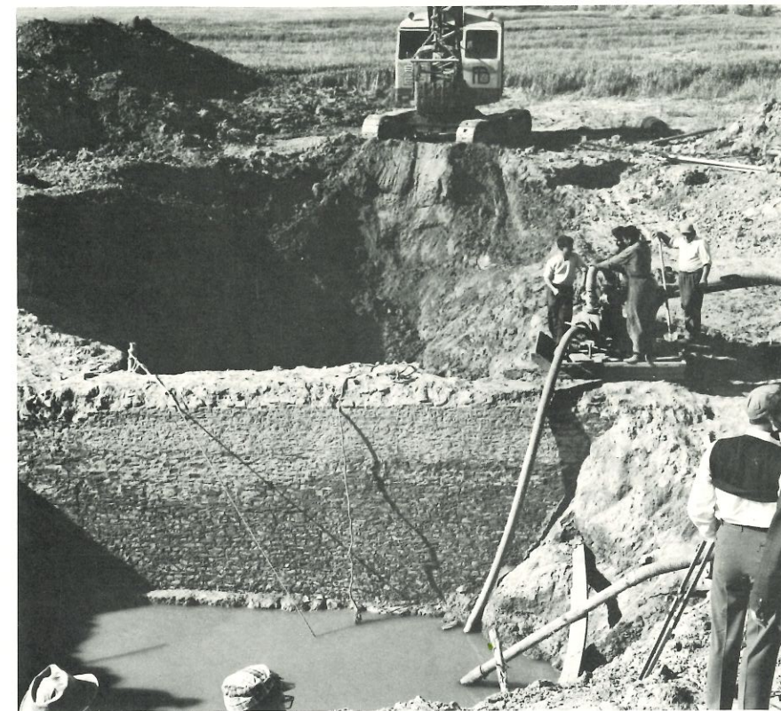
Figure Five. Excavation of the Long Wall with a drag line shovel. As two pumps try to keep abreast of the ground water rising south of the wall Greek foundations begin to appear under the Roman wall.
