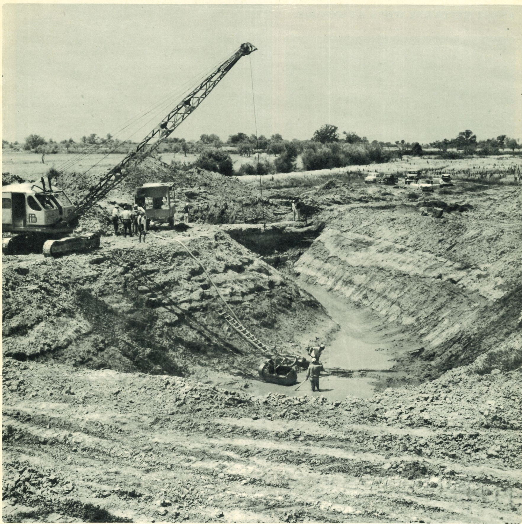
FIG. 2. THE DRAG-LINE CLEARING THE 4TH-CENTURY GREEK STRUCTURE NORTH OF THE LONG WALL. ELECTRIC PUMPS ARE DRIVEN BY A GENERATOR IN THE TRUCK TRAILER.
