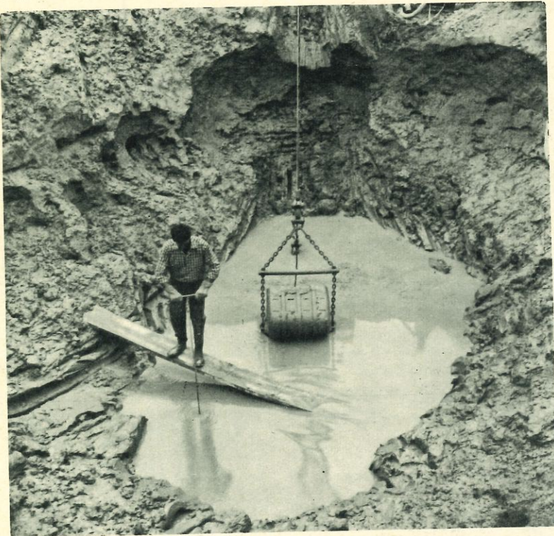
FIG. 3. "THE SPILO," A THIN METAL ROD CAPPED WITH A T-SHAPED SECTION, BEING USED TO "FEEL" FOR BURIED WALLS IN SECTION B.
